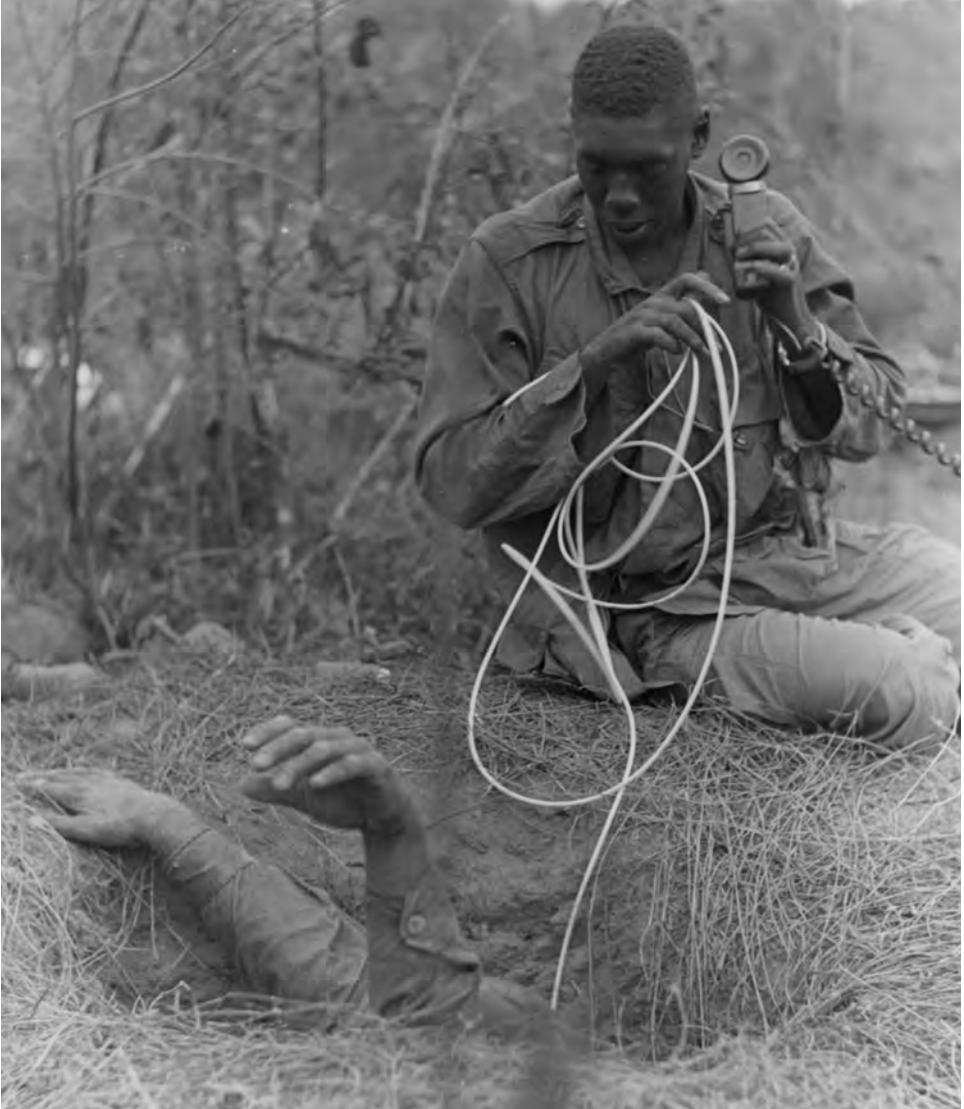
Detonating cord used to initiate an explosive charge is lowered into a tunnel by troops of the 173d Engineer Company, 173d Airborne Brigade, during Operation CEDAR FALLS.
